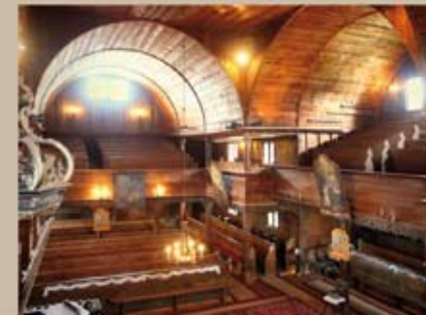
Wooden column architecture and slab barrel vaults – Hronsek
